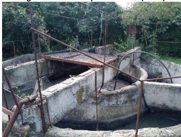
Figura 4-10: Deznisipator circular (SEAU)
