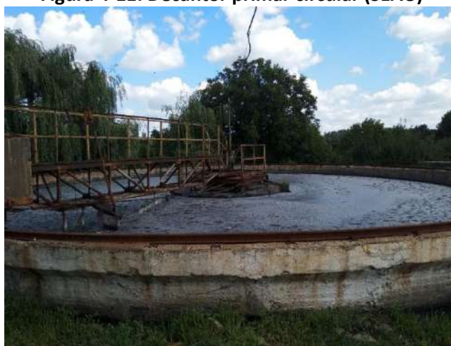
Figura 4-11: Decantor primar circular (SEAU)
