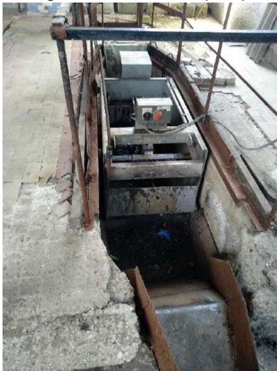
Figura 4-9: Grătar mecanic (SEAU)
