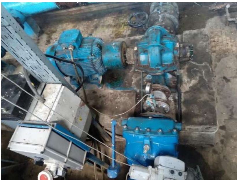
Figura 3-17: Pompa WEIR SDCD 150/200 (SP-03)
